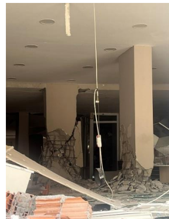
Column failure
