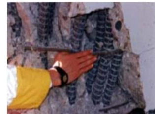
Photo_5: Failure of Column due to inadequate shear reinforcement. These photos are taken from different earthquake events. Collapse of heavily loaded columns may cause collapse of the building. These structures were built with the original earthquake-resistant philosophy that was collapse prevention.
