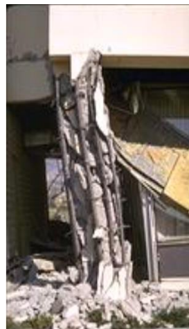
Photo_5: Failure of Column due to inadequate shear reinforcement. These photos are taken from different earthquake events. Collapse of heavily loaded columns may cause collapse of the building. These structures were built with the original earthquake-resistant philosophy that was collapse prevention.
