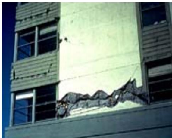
Photo_4: Close-up of the failure of one of the shear walls in a building showing incipient types of failure at the construction joints due to poor workmanship at the joints. The failure of this particular wall did not occur at the construction joint, and it was attributed to lack of adequate axial-flexural capacity. Note the lack of any extra reinforcement at the edge of the shear walls.
