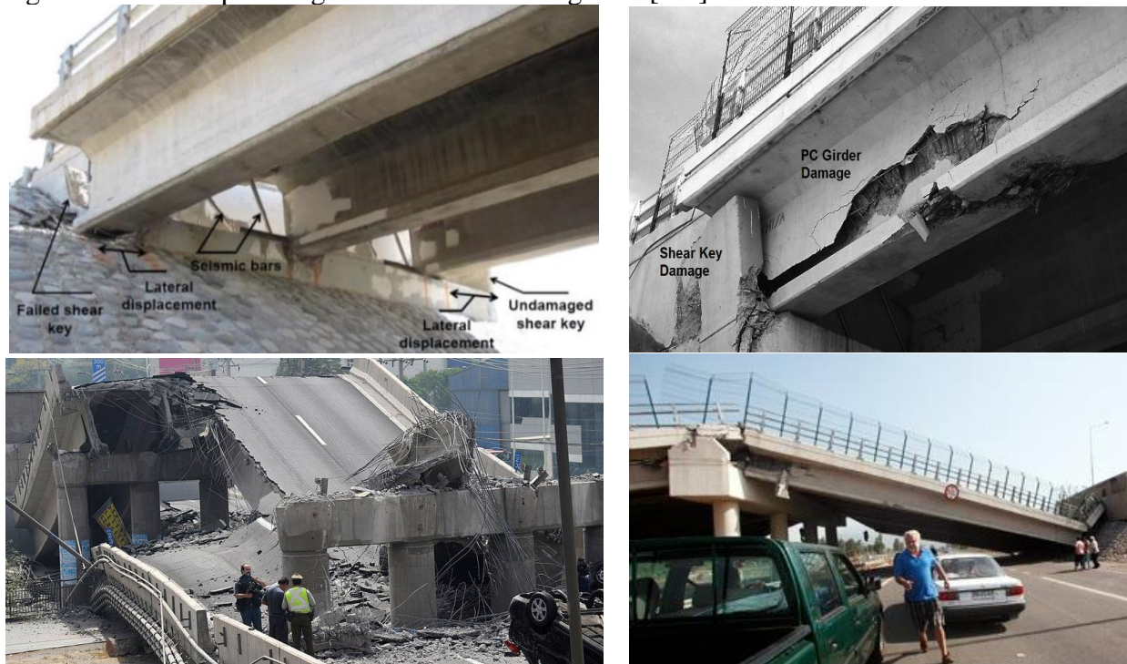
Figure.1. - Damage observed in highway bridges after the 2010 Maule earthquake
