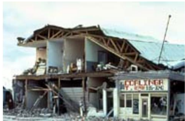
Photo 2: The second story 8-in. unreinforced solid brick masonry walls of this commercial building in Coalinga collapsed during the 1983 Coalinga Earthquake because of inadequate tying at the floor, roof, and transverse walls.
