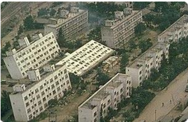
Photo_8: Collapse of Apartment Buildings due to soil liquefaction during the 1964 Niigata earthquake.
