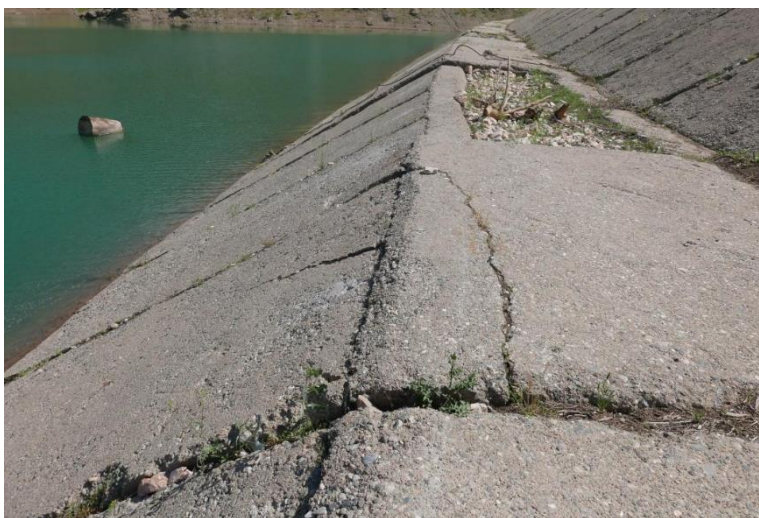
Figure 5. – Cracks and subsidence of reinforced concrete fastenings from the upstream side
