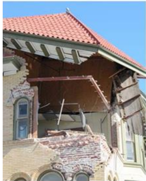
Photo_3a and Photo_3b: Overview and detail of supporting column and walls at the top corner of a Commercial Building during the 2014 South Napa Earthquake. Note the remaining epoxy anchors between the diaphragm and brick walls.
