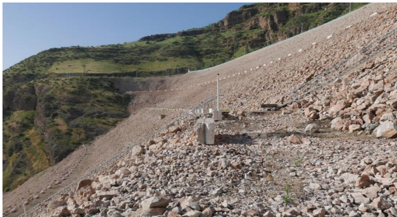
Figure 4. – Local traces of reshaping of the downstream slope as a result of compaction and sliding of rockfill from the downstream side
