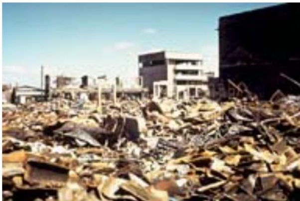
Photo 1: View of downtown Managua City, Nicaragua, after the 1972 Managua Earthquake. The debris is from the complete collapse of unreinforced masonry and adobe buildings.
