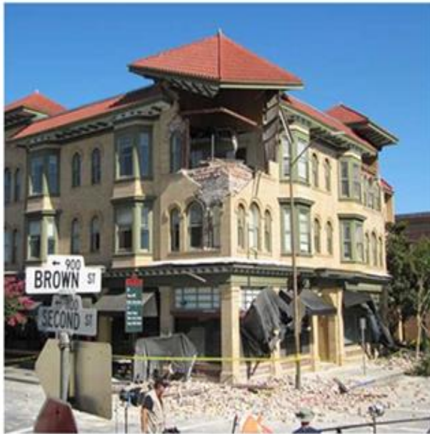
Photo_3a and Photo_3b: Overview and detail of supporting column and walls at the top corner of a Commercial Building during the 2014 South Napa Earthquake. Note the remaining epoxy anchors between the diaphragm and brick walls.
